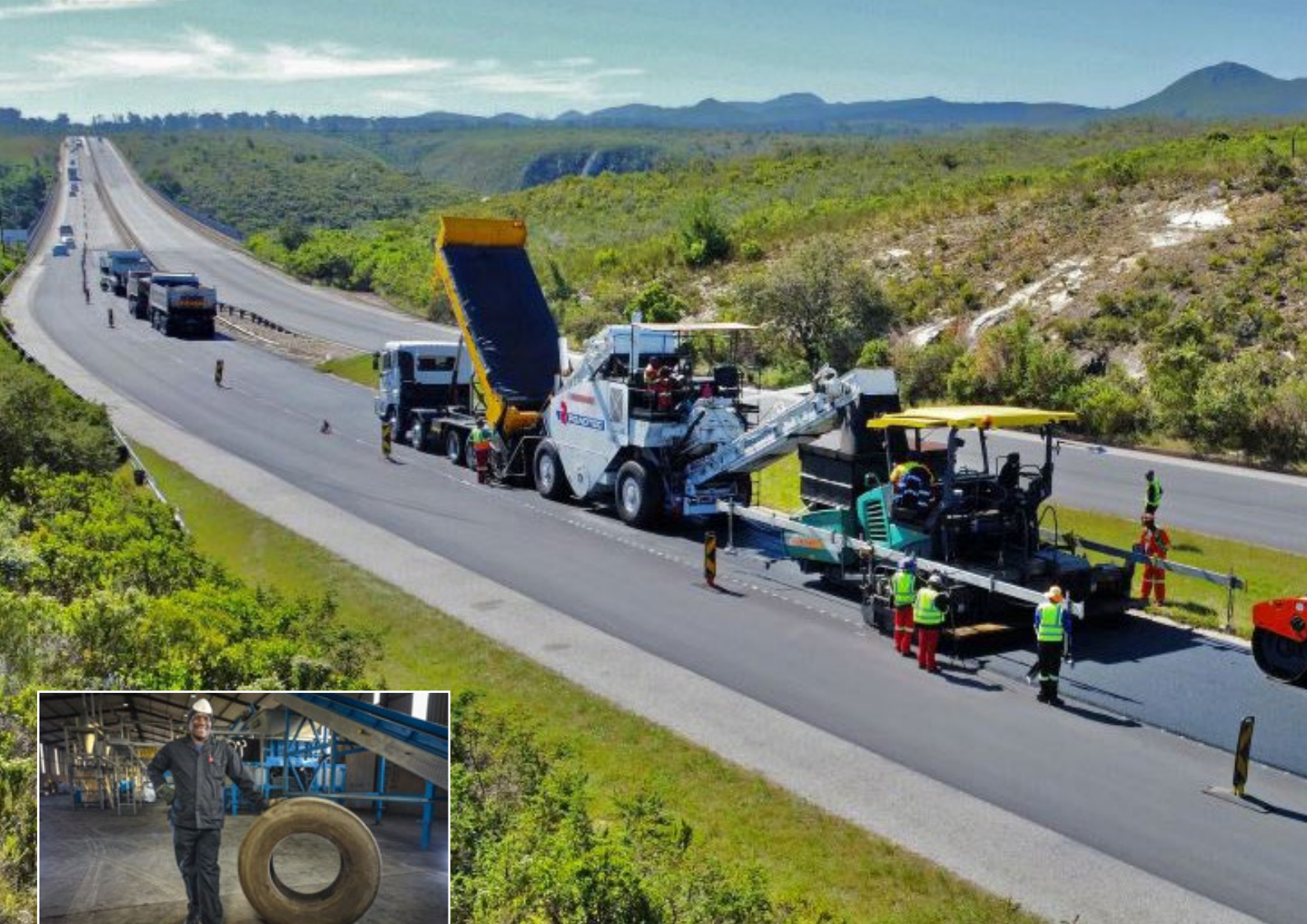
▲ Rubber bitumen in a typical asphalt overlay application on the N2 near Gamtoos River.
