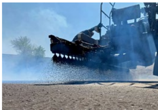
▲ Rubber bitumen being applied for a spray seal application.
