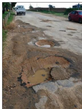
▲ These pictures show the extent of damaged roads around the Johannesburg area. In some provinces, roads have been like this for ages due to maintenance neglect. Tyre impact fractures are the danger here as can be seen in the photograph on the left – taken from inside a pothole - which clearly shows what a tyre has to go through when it hits a pothole. Hit it at speed and you could end up dead from a blow-out.
